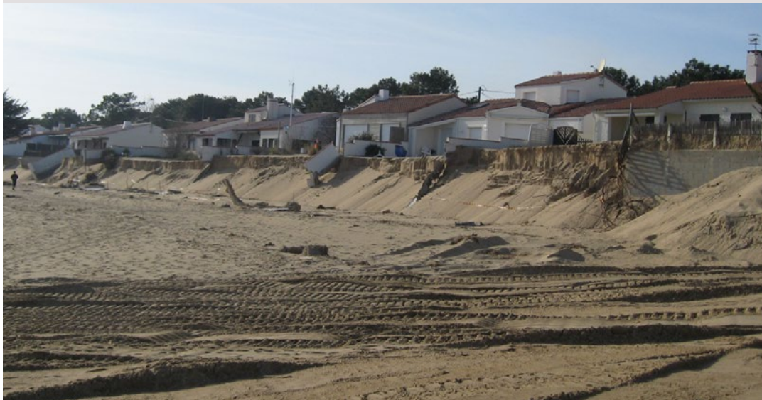
Figure 2 – Retreat of the dune at La Tranche-sur-Mer, Vendée, following storm Xynthia – March 2010 (Photo: © Bruno BERENGER, Cerema)
